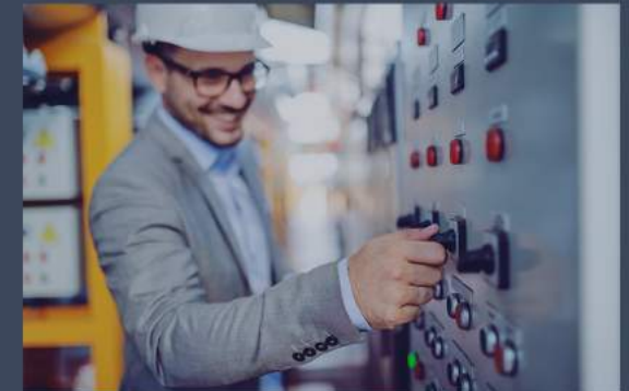
Experience uninterrupted power supply
